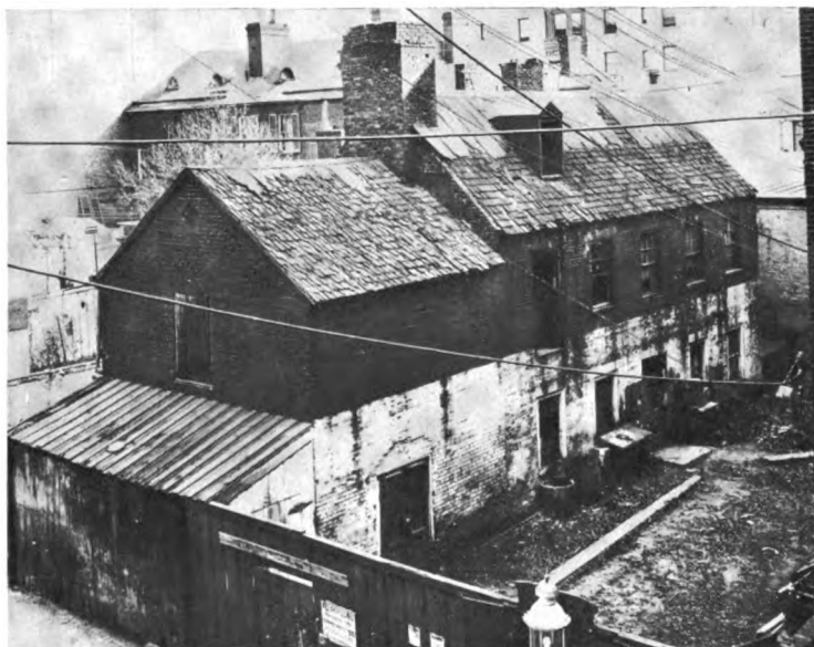
REAR 1417 F STREET, N. W., ORIGINALLY KNOWN AS THE LITTLE HOTEL.
